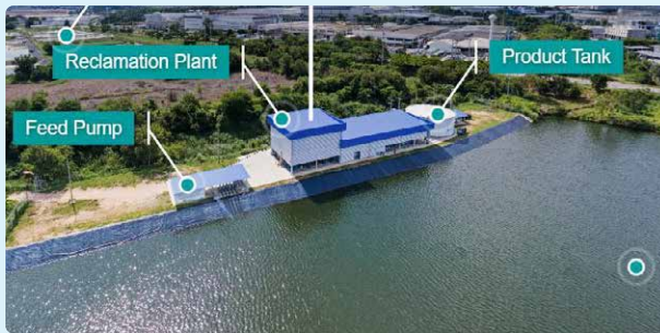
Reclamation Plant at ESIE
