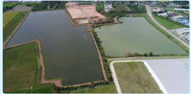
Water Reservoir Construction Project at WHA SIL
