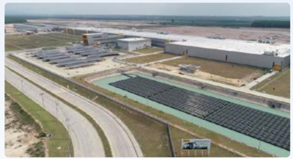
Floating Solar System
