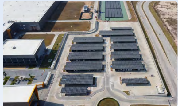
Solar Car Park
