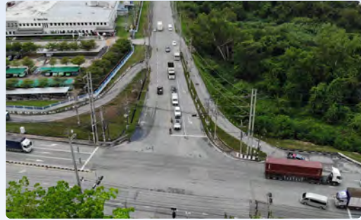
Picture 2: Expansions traffic lane in E-6 Road by expanding road 2 lanes to 4 lanes, thus increasing traffic flow.
