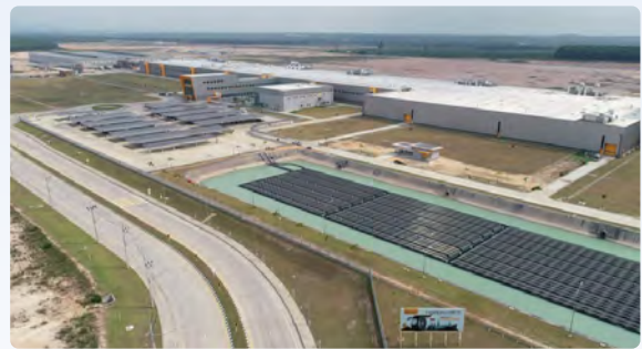
Floating Solar System
